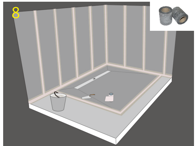
8. All butt joints are sealed with waterproof sealing tape using tile adhesive.
