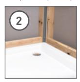
The first profile, which normally starts with an Internal Corner or End Cap, should be fixed to the wall or end grounds with countersunk screws, or adhesive and a bead of silicone sealant applied to the channel
