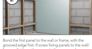
Bond the first panel to the wall or frame, with the grooved edge first. If screw fixing panels to the wall/frame, pilot bore the recess in the groove where screws are to be located. Failure to pilot bore may result in the panel's joint splitting). Pack between back of panel and wall as necessary to avoid distortion to the tongue & groove joint when screw fixing and to ensure that it is true and plumb.
