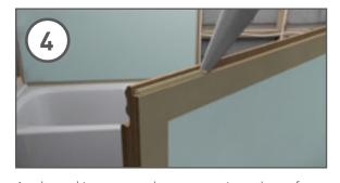
Apply masking tape to the two meeting edges of the decorative face to protect the laminate face. Apply a narrow bead (2-3mm) of silicone sealant to the front shoulder of the tongue. Note: Using too much silicone sealant will affect the tightness of the tongue & groove joint. Using too little may affect water-tightness.
