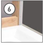
Apply high grab adhesive to the reverse of the **Dura**panel® angle into the first profile and push firmly against the wall.
