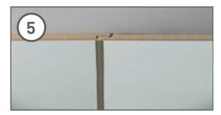
Slide the tongue of the next panel into the groove. Ensure the tongue is fully inserted into the groove. Excess sealant should squeeze out and this should be wiped clean with a cloth.
